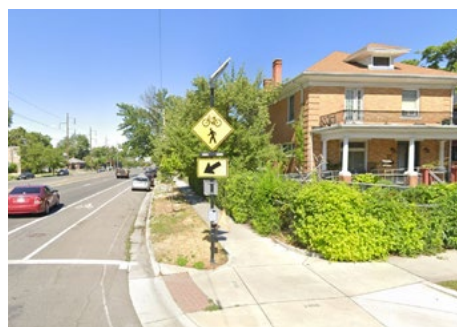
RRFB Signage & flashing beacon in Salt Lake City, UT Source: Google Earth
