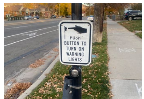
RRFB push button signage
